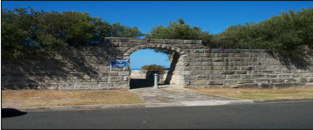
Freshwater View Reserve – Pavilion St Queenscliff
